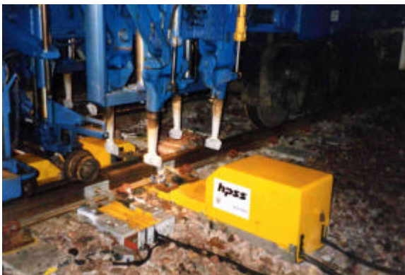
Machine Tamping of HPSS (Nunhead Junction - November 2000)
