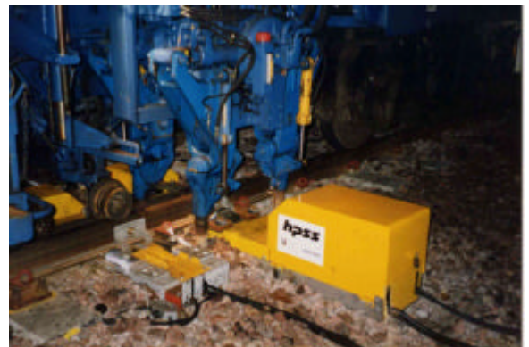
Machine Tamping of HPSS (Nunhead Junction - November 2000)
