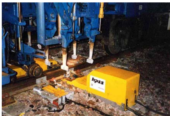
Machine Tamping of HPSS (Nunhead Junction - November 2000)
