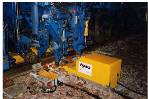
Machine Tamping of HPSS (Nunhead Junction - November 2000)
